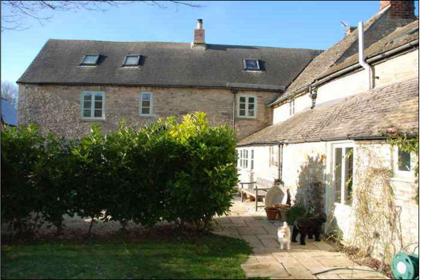
Rear aspects of the extended farmhouse
